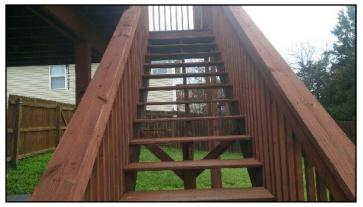
16. Condition: • Spindles nailed on.Implication(s): Nailed spindles tend to pull away.Task: Improve/Use exterior screws
