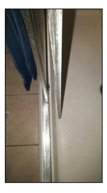
**55.** Condition: • The protective flange, known as an escutcheon, is not properly sealed or caulk at the shower stall assembly.
