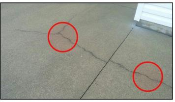
**20. Condition:** • The Patio expansion joints are not sealed with suitable materials to shed water. Implication: Water will infiltrate the expansion joints and cause cracks due to expansion of the water inside the joints. Task: Caulk is advised.
